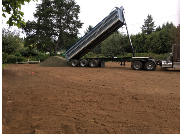
Adding concrete sand
