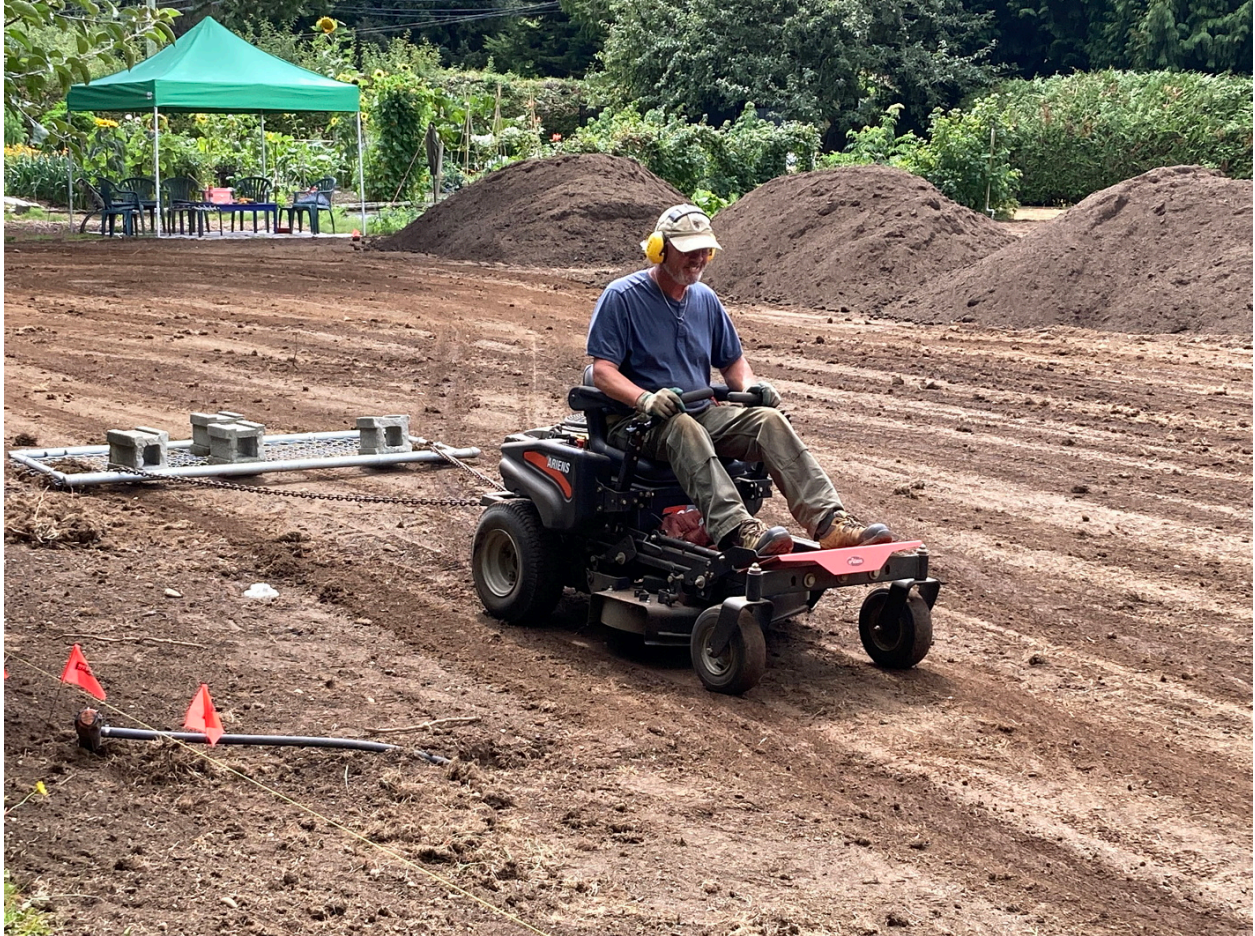
Michael Dowling grades the subgrade at the Happy Valley Croquet Club
